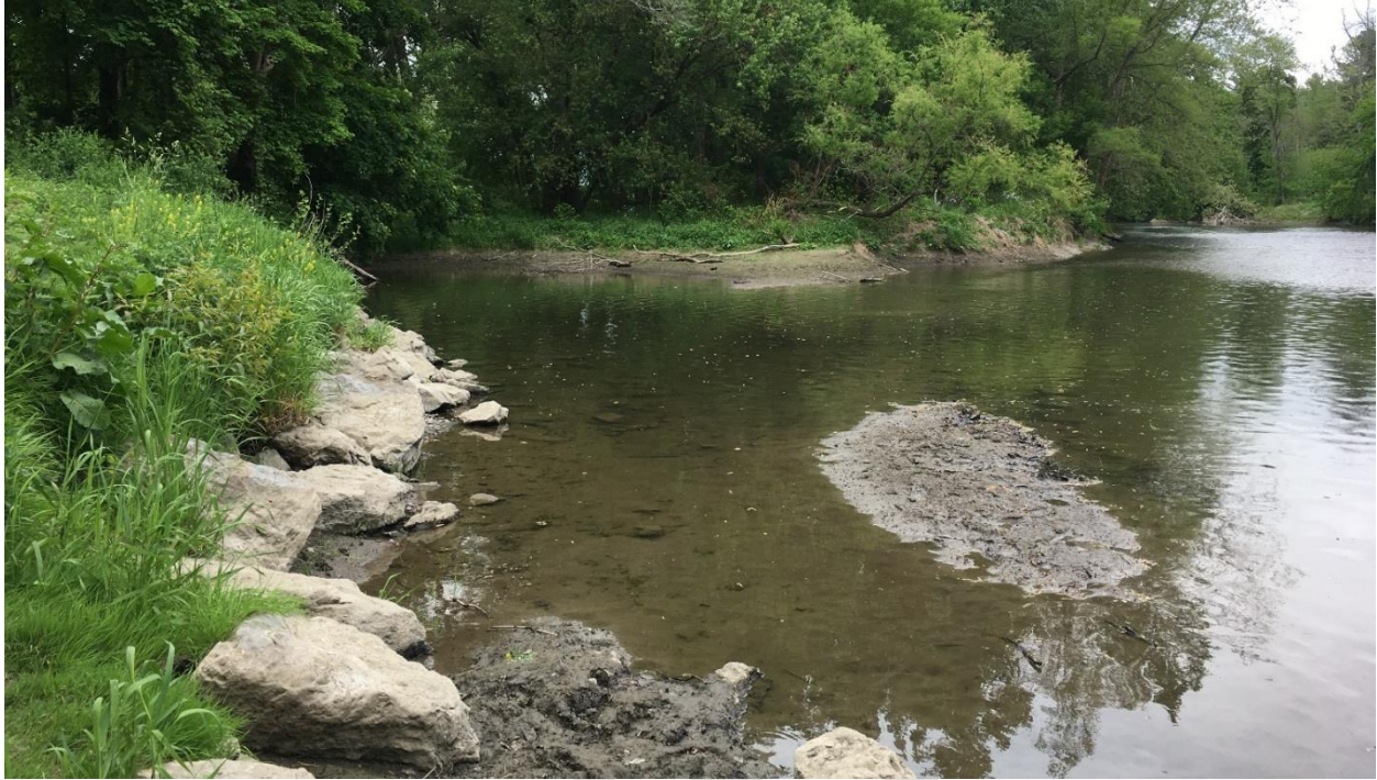
Figure 9: Riprap with steep edge to the south of the inlet.
